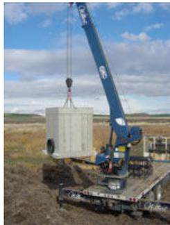
Installed within the preconstructed levee, the precast concrete structure, which weighs approximately 10 tons, is lowered into position. A culvert runs through the dike to provide an outlet for the water. Stop logs, consisting of oak boards that measure 5 feet wide by 3 inches thick and 6 inches tall, rest between the 6-inch-thick precast walls of the structure. Depending on the desired water level, stacked stop logs can be added and removed to control the amount of water that will be
