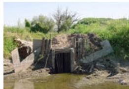
At first, three materials were considered for the water control structures: galvanized steel, cast-in-place concrete and precast concrete. Steel was ruled out for the water control structures because of the extensive welding required and need for long-term durability. Initially, Ducks Unlimited considered the use of
